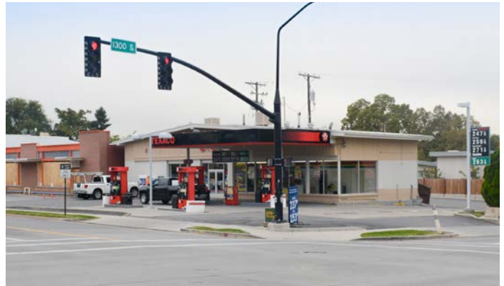
The above photo is a view of the south-west corner of the 1300 S & 2100 East node.
