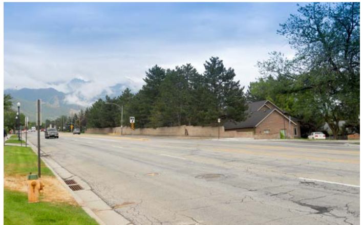
Parley's Way functions as a main access route into and out of the east Sugar House community. Its wide, unconstrained travel lanes can result in high vehicle speeds.
