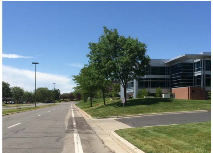
Research Park developed as a car oriented, suburban style office park and in many places lacks the sidewalks and bike paths that would encourage active circulation in the park and to other regional facilities.
